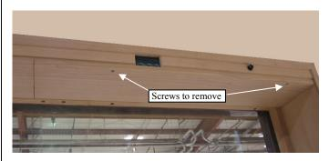
Step 3: Remove cover of standard junction box only, as shown.
